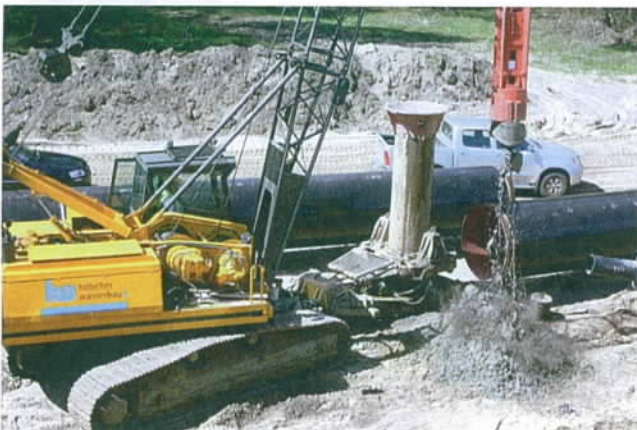
Figure 3. Casing drilling rig.
